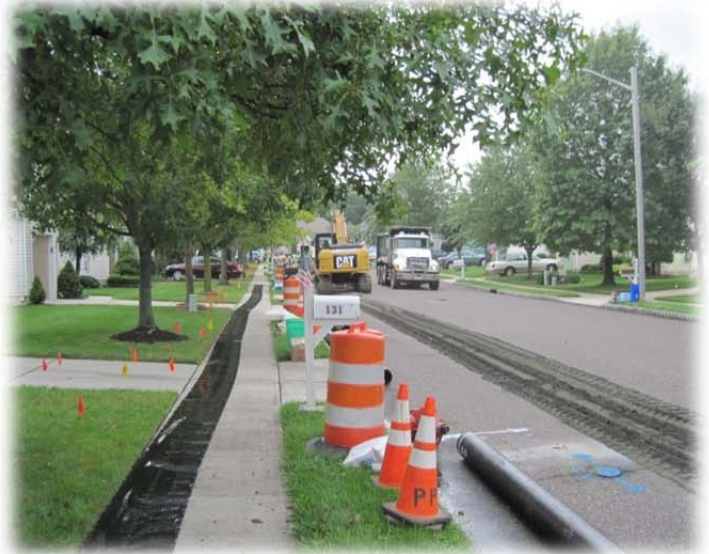
Preparation for Indigo Drive water main replacement
