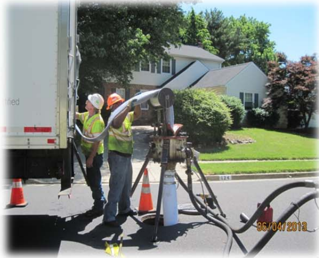
Sanitary sewer main rehabilitation project
