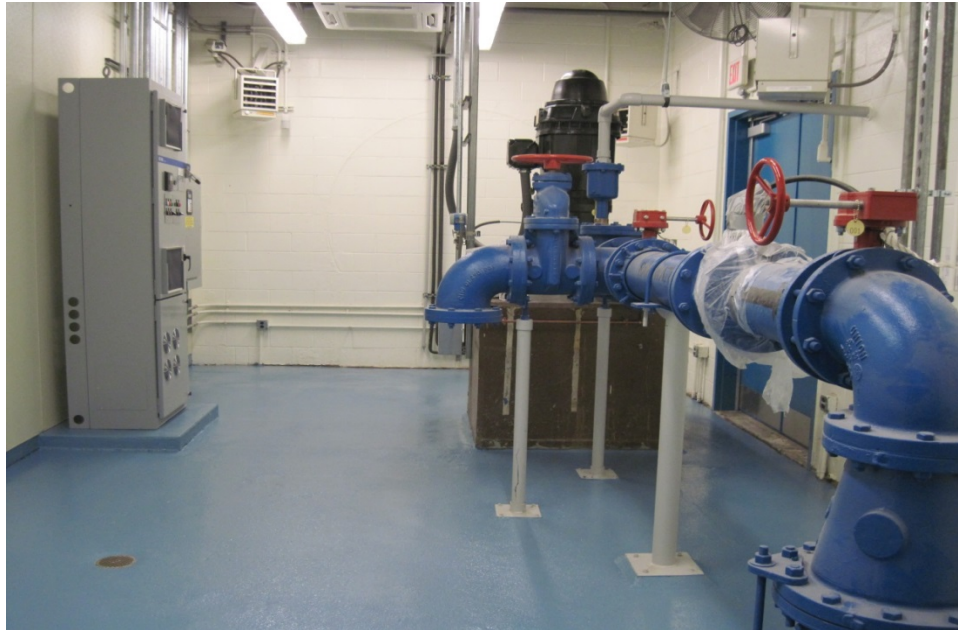
Well #4 – Equipment and well improvements
