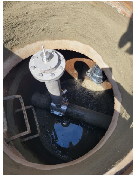
New Air Release Valve Installed
