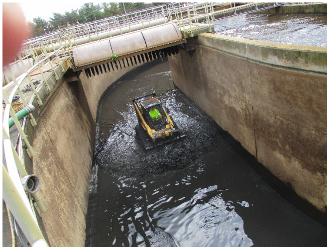
Removal of Heavy Sludge to Prepare for Concrete Repairs
