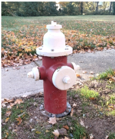
A Repaired Fire Hydrant
