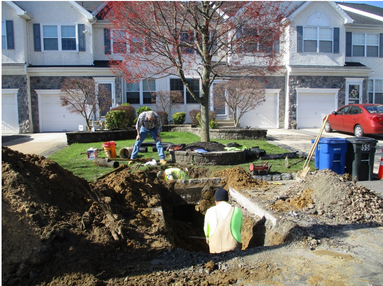
Installing Replacement Water Service Connections
