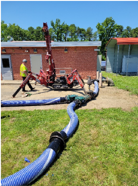
Replacing Valves in the Ramblewood Pump Station (the largest of the Authority's 41 pump stations)
