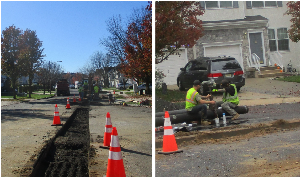
Water Main Replacement in Chapel Hill Rd
