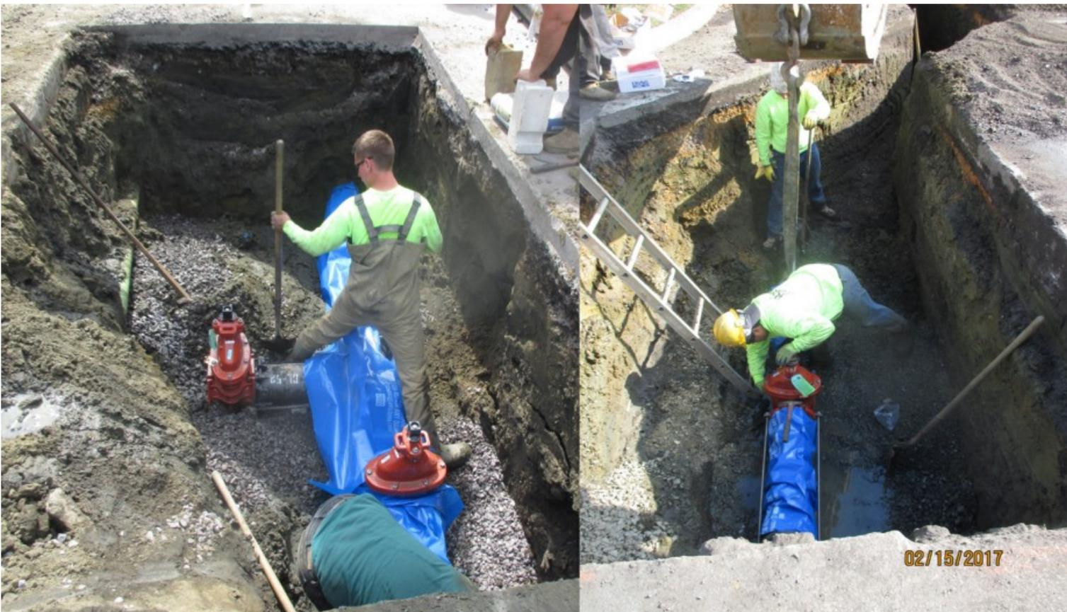
Left: RTW Contractors, Inc. of Southampton, NJ installs replacement water piping in Grant Road; Right: S. St. Andrews Drive—installation of new water main wrapped in plastic by RTW Contractors, Inc.
